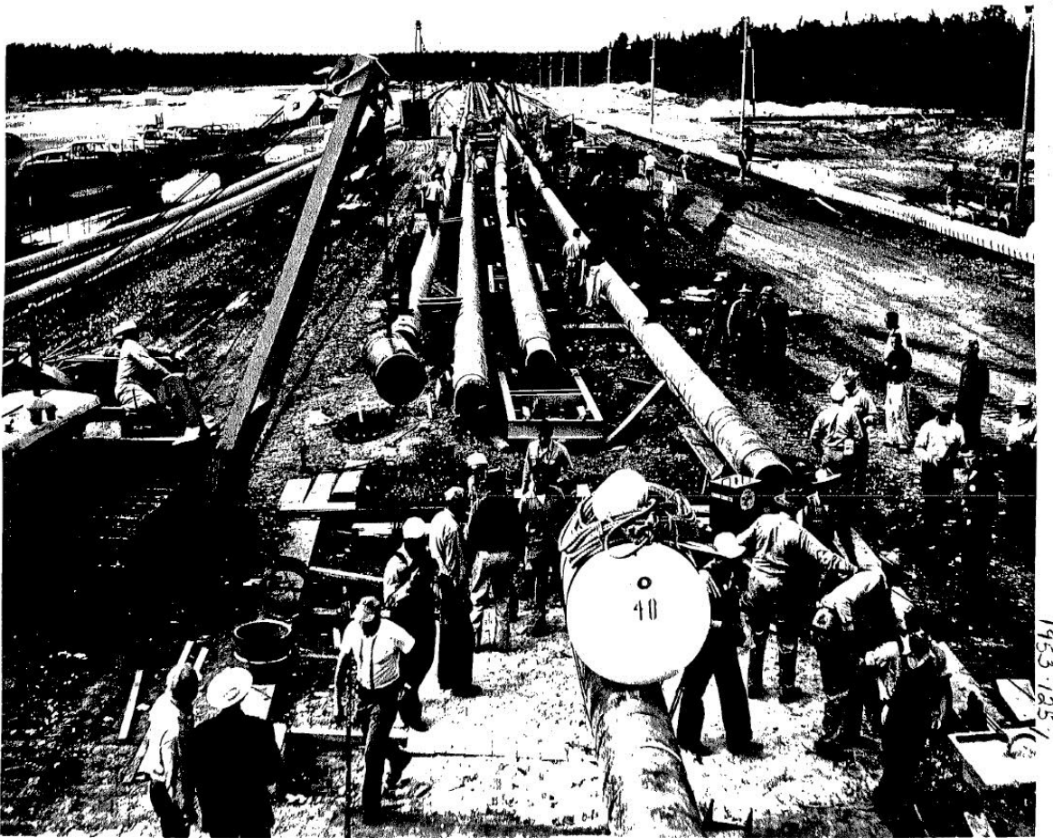
Figure 29. 1953 Photograph Showing Curvature of Pipe String as it is Moved onto the Launch Way Using a Crane
