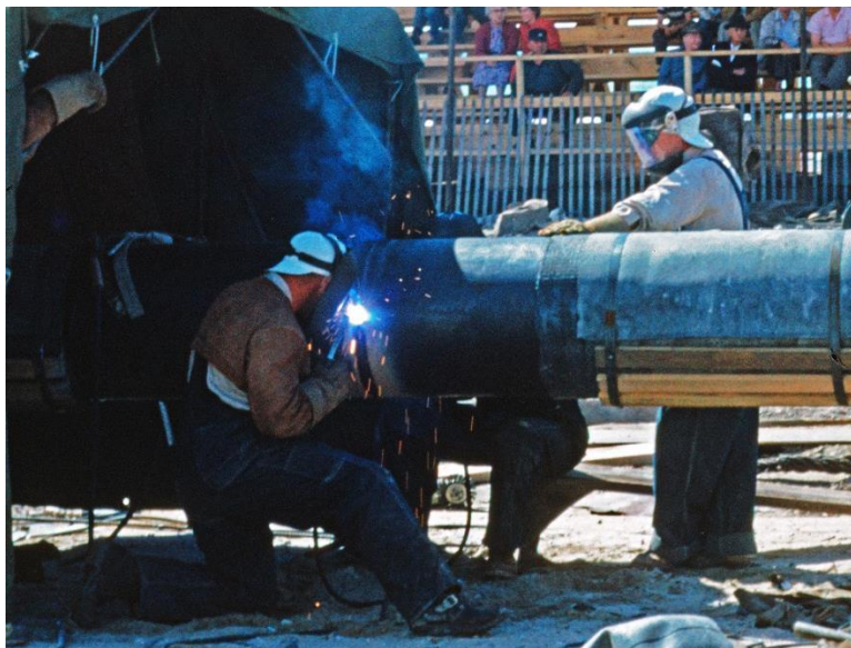
Figure 5. Trudgen Photo of Pipe String Assembly Welding (00010370005.tif)
