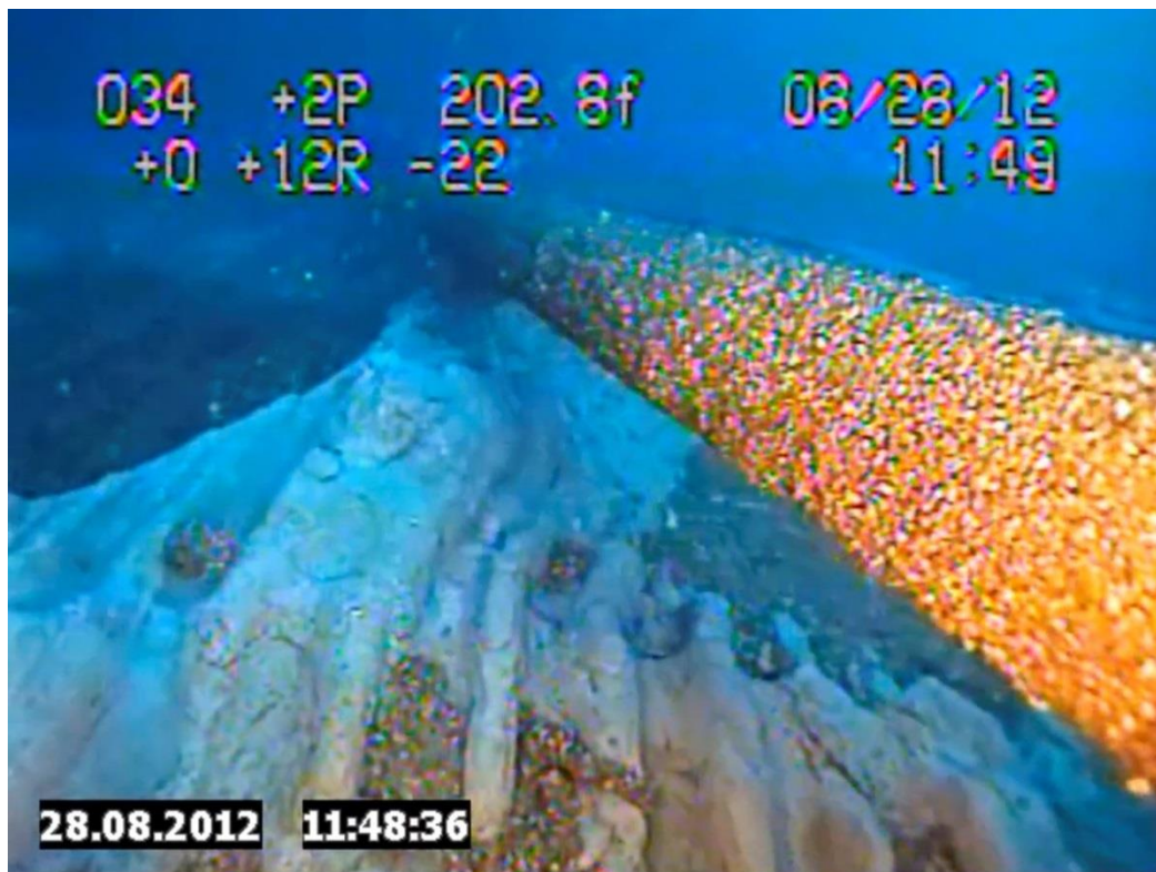
Figure 19. Photo of Unsupported Span Clipped from Enbridge Underwater Inspection Video from the 2012 Inspection (East Leg, ~203 feet water depth)
