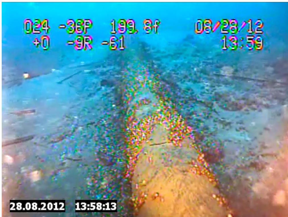
Figure 11. True Color Photo Clipped from Enbridge 2012 Underwater Inspection Video of the East Line Taken on 8/28/2012 at 13:58:13 Showing Missing and Disbonded Coating and Rusty Coloration of Pipe with Apparent Pitting Corrosion
