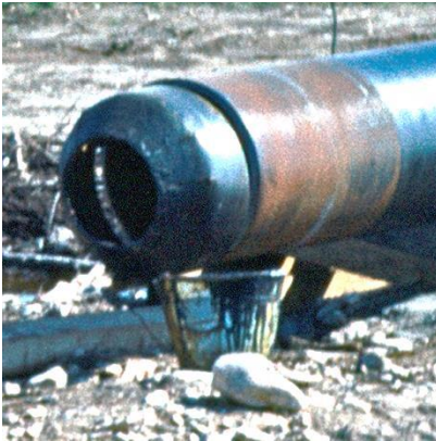
Figure 3. Detail Enlarged from Trudgen Photo of Pipe Wrapping Machine Showing Wrapped Pipe (00010370012.tif)
