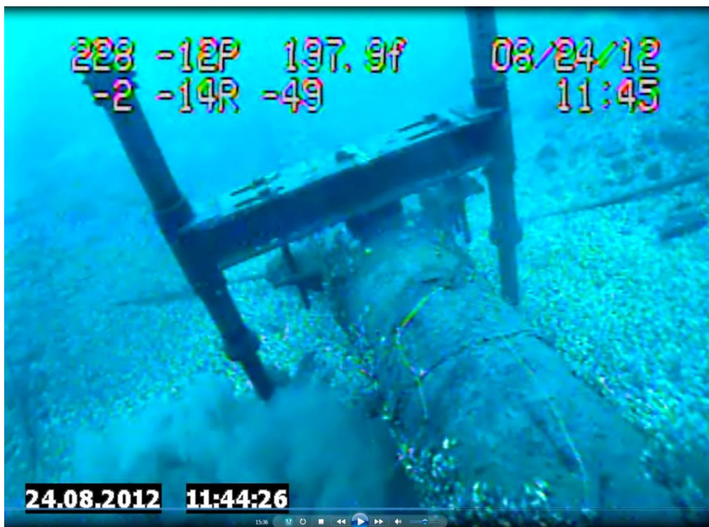
Figure 8. Photo Clipped from Enbridge 2012 Underwater Inspection Video of the East Line Taken on 8/24/2012 at 11:44:26 Showing Missing and Disbonded Coating
